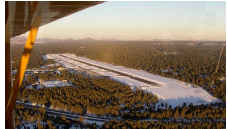
Flagstaff Airport from visual approach to rwy 3. Rwy is 2.700 m; rwy 21 is ILS-equipped.
