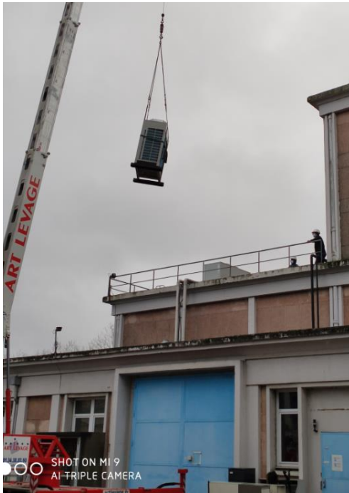
The cold group is installed on the roof of the hall
