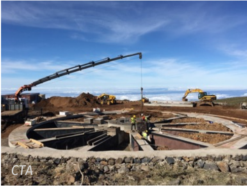
January 2017: Completion of foundation
