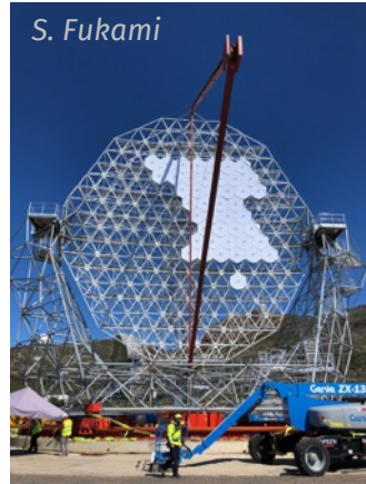
April 2018: Mirror installation
